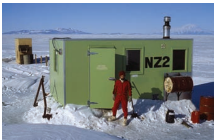
Figure 4. A portable laboratory with a 7.5 kVA diesel power generator was set up over a fishing hole drilled through the 2 m thick ice cover on the Ross Sea, Antarctica. The hut was heated to prevent the seawater from re-freezing and to allow the researchers to conduct physiological experiments.
