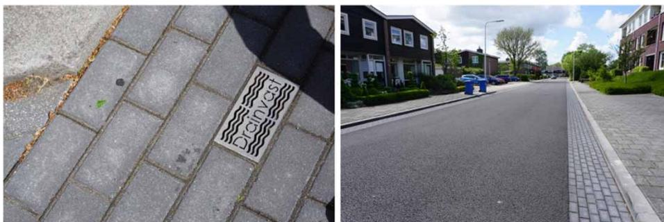
**Figure 6** | Case #33 has been assigned the root cause *Incomplete knowledge* about the internal technical processes. The pavers were separated by joints filled with a permeable material, allowing water to infiltrate. Even after a small rainfall event, however, water remained ponding for at least 1 h. As such, it was thought that the permeable material had become clogged, leading to a malfunction of the SUDS.
