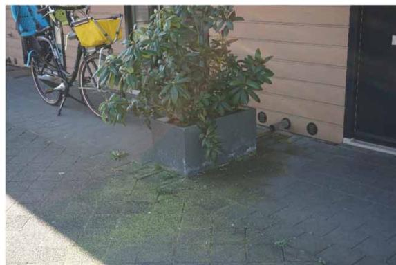
**Figure 7** | Case #8 has been assigned the root cause actual use of SUDS. A flowerpot was placed in front of a dwelling's water outlet, preventing water to be discharged properly.
