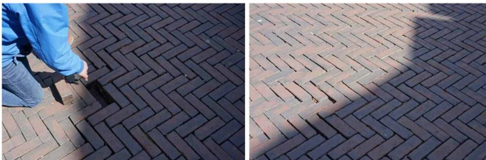
**Figure 5** | Case #29 has been assigned the root cause *Incomplete knowledge* about the interactions of SUDS with other urban systems. Due to the impact of cars as well as street sweeping, the joints of the permeable pavement bricks vanished. This decreased the overall performance of the SUDS, i.e., the stability of the road surface.
