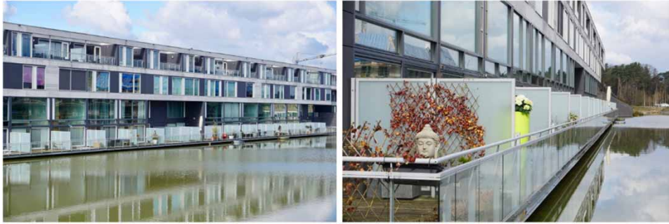
Figure 4 | Case #60 has been assigned the root cause poor communication between different actors. Due to lacking communication between the architect and the municipality, the houses were built only 0.15 m from the water level. This minimized the storage capacity of the surface water, while the water was initially designed as a storm water detention pond with a freeboard of 0.70 m.
