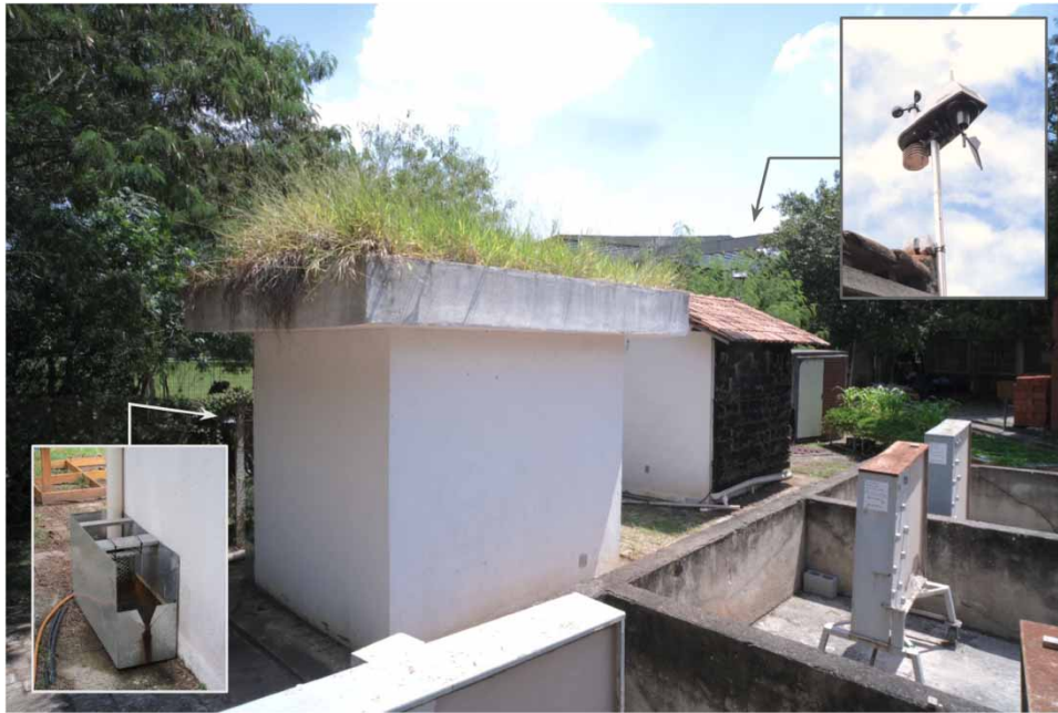
Figure 6 | Vegetated roof building prototype and CT roof building prototype, highlighting the triangular-notch weir tank with the ultrasonic sensor and the Vantage Vue weather station. Source : the authors.
