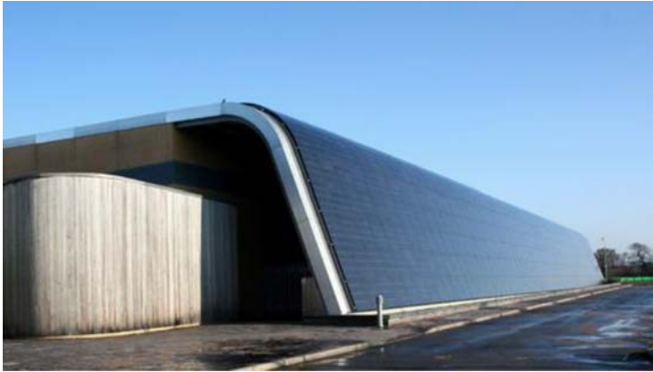
Figure 1.4 The 85 kW p thin film PV façade at the OpTIC building in St Asaph, North Wales, generating 70 MWh of electricity per year. The modules are Shell ST36 CIS and the total array area is 1176 m 2 .
