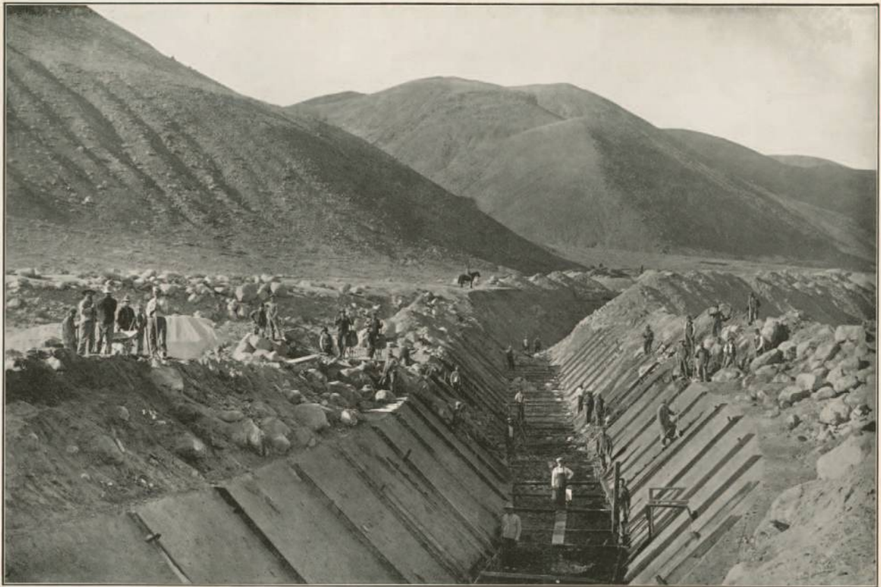
CONSTRUCTION OF OPEN LINED CANAL IN OWENS VALLEY
