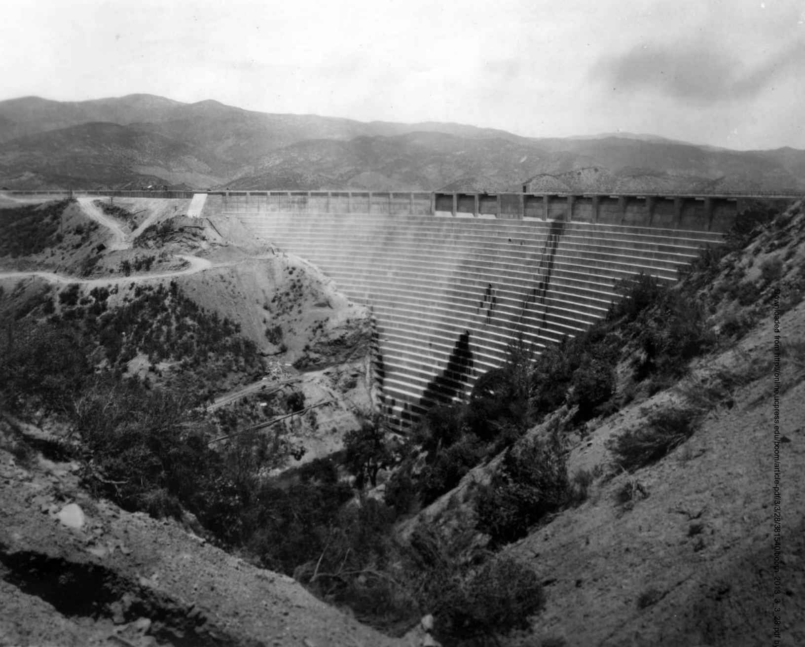
St. Francis Dam beginning to leak. COURTESY OF THE LOS ANGELES PUBLIC LIBRARY PHOTO COLLECTION.
