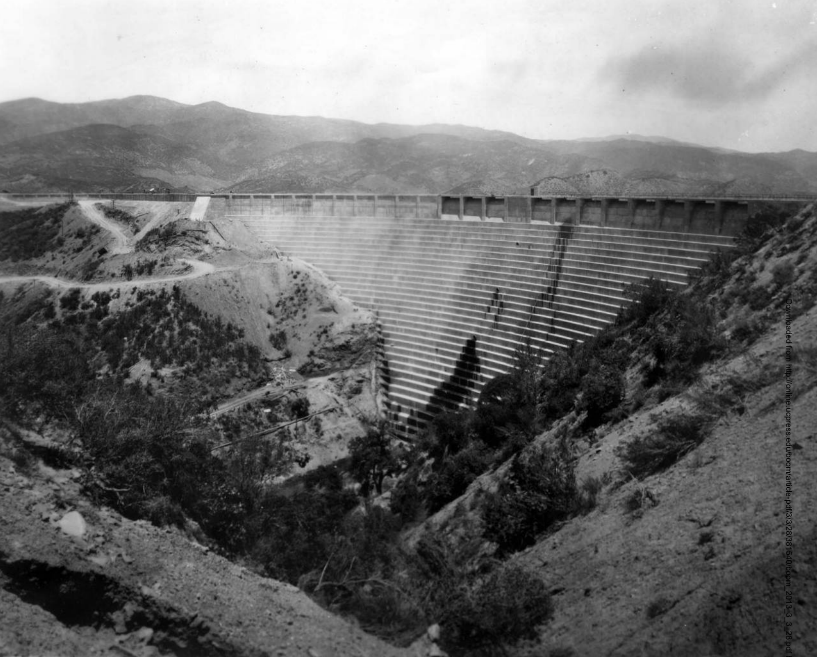
St. Francis Dam beginning to leak. COURTESY OF THE LOS ANGELES PUBLIC LIBRARY PHOTO COLLECTION.
