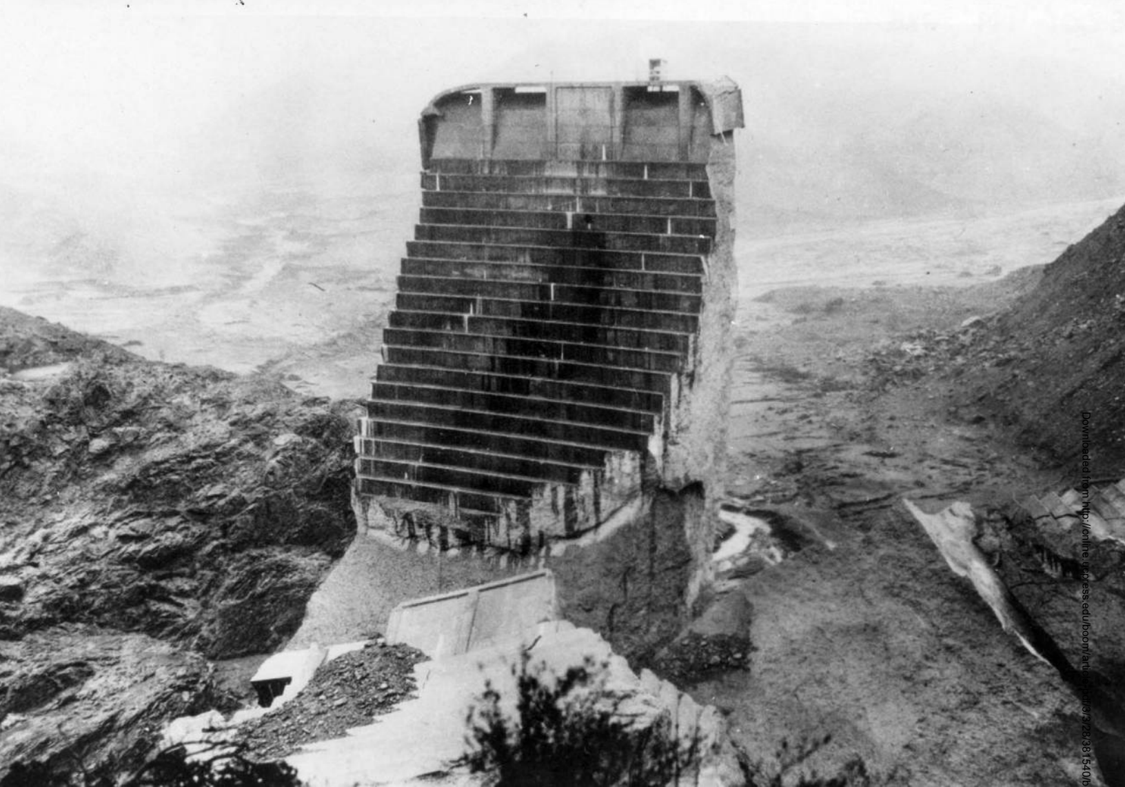
The remains of St. Francis Dam. COURTESY OF THE LOS ANGELES PUBLIC LIBRARY PHOTO COLLECTION.
