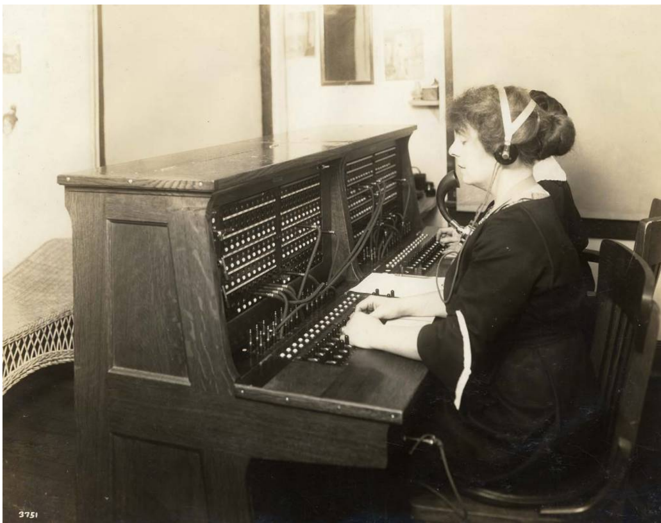
Telephone switchboard in service building at the Panama-Pacific International Exposition. COURTESY SAN FRANCISCO PUBLIC LIBRARY.
