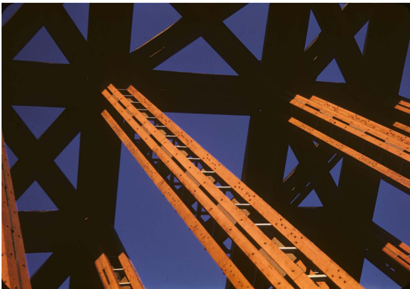
Detail of construction of the “nave” of the Federal Building. From the Visual Resources Center, University of California, Berkeley.
