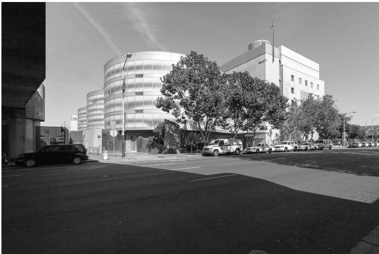
San Francisco County Jail #1. Photograph by Taiyo Watanabe.
