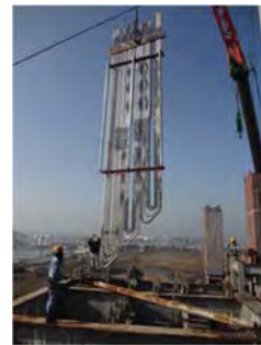
Fig. 16 Lifting of 3 rd path of 700°C SH (Courtesy of IHI)
