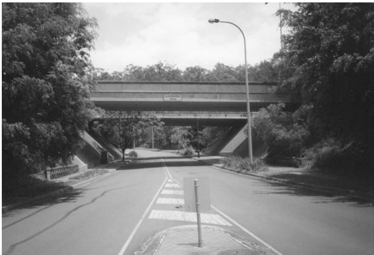
Figure 12. Road underpass under the Gateway Freeway between Belmont Hills and Mt Petrie. The forest of Belmont Hills is visible in the background.
