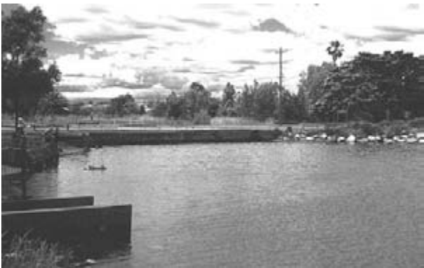
Figure 7. The view from pond 1 to pond 2 at Barton Street in the Rockdale wetland area shows the water constriction due to the causeway. The stormwater drain on the left is visible with residential house roofs and backyard trees in the background.
