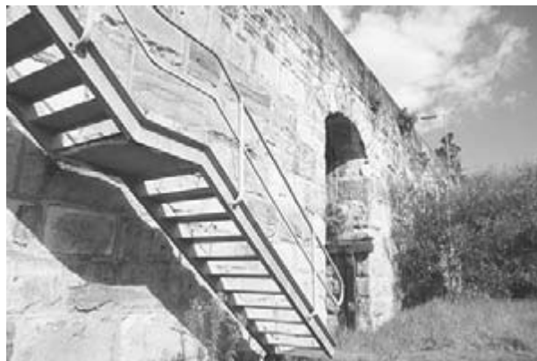
Photo 2. The Coal Loader at Balls Head, North Sydney, provides a secure roost for several hundred Large Bent-wing Bats.
