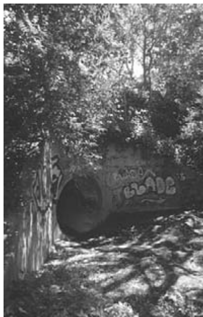
Photo 4. Up to 1000 Large Bent-wing Bats use this stormwater drain.
