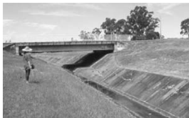
Before restoration - Clear Paddock creek in 1995 - a bleak concrete-lined storm water channel. Photo: M. Crawford
