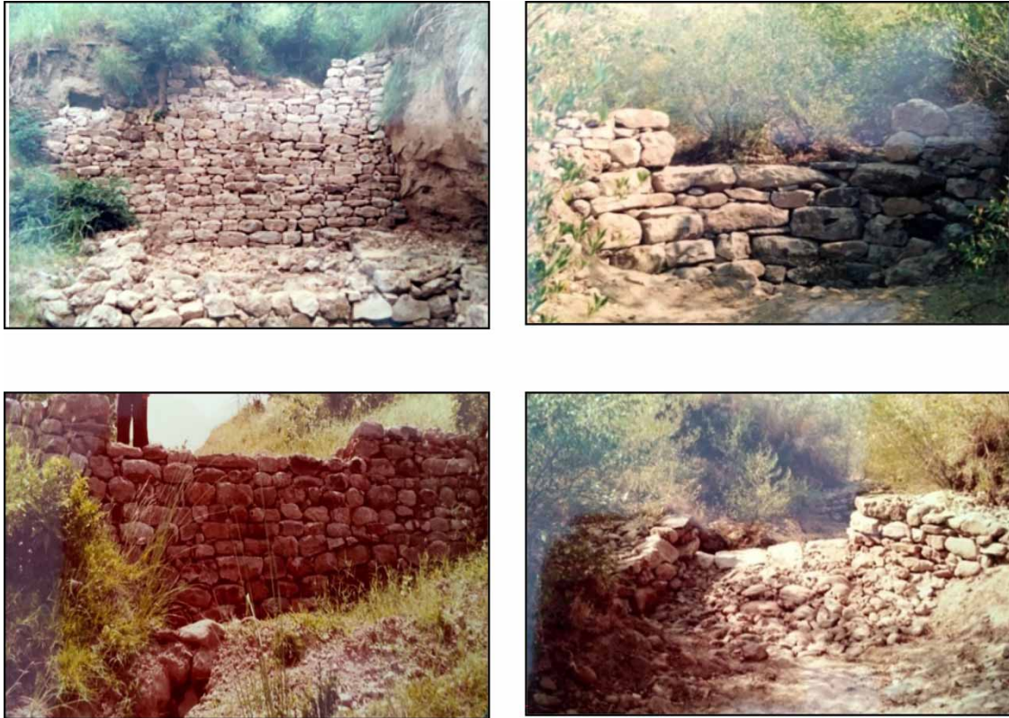
Figure 2 | Check dams at the drainage line of microwatershed-I.
