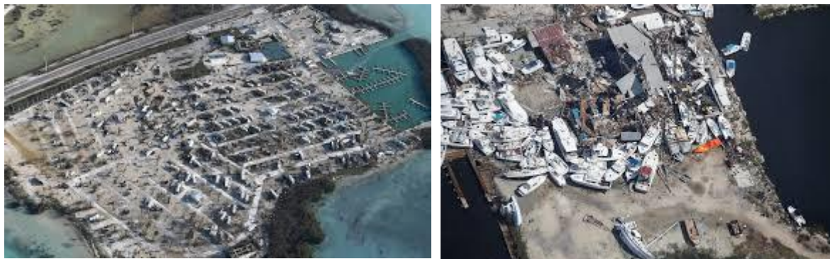
Figure 4. Examples of damage caused by Hurricane Irma in Key West (source: aol.com )
