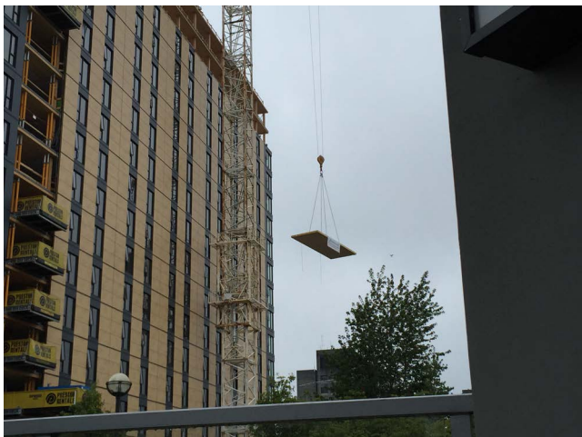
A panel is being lifted into place during construction of the 18-story Brock Commons Tallwood House student residence at The University of British Columbia.
