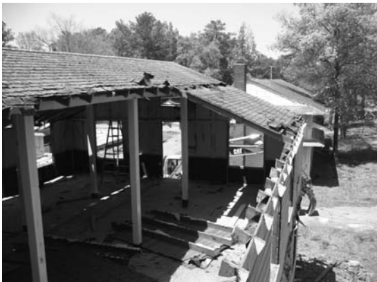
PHOTOGRAPH 2. Roof panelization
