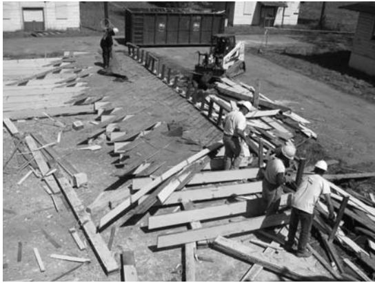
PHOTOGRAPH 5. Hand disassembly of dropped second floor
