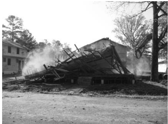
PHOTOGRAPH 4. “Dropping” second floor by collapsing onto first floor
