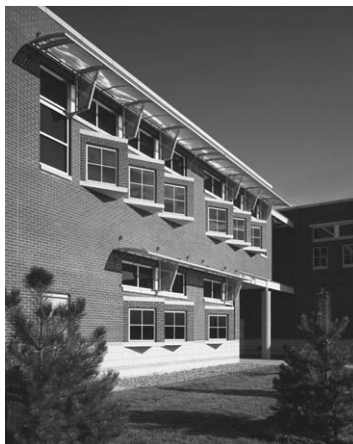
West classrooms elevation. Note how windows are turned 30 degrees off true west.
