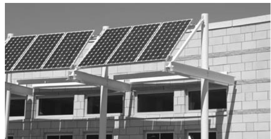
Photovoltaics shading office windows.
