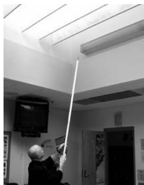
FIGURE 6. Manually operated vertical blinds on the roof monitor windows can be drawn to darken rooms for audio-visual presentations.
