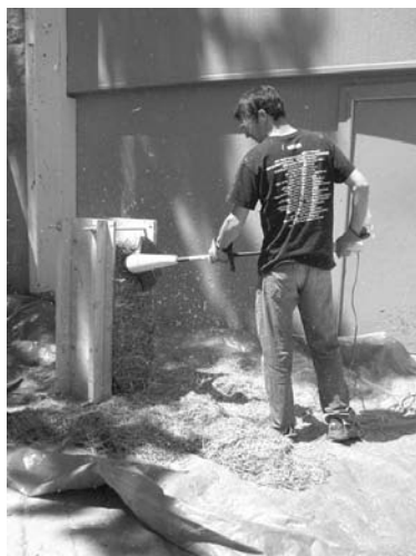
(b) Trimming bale in jig.
