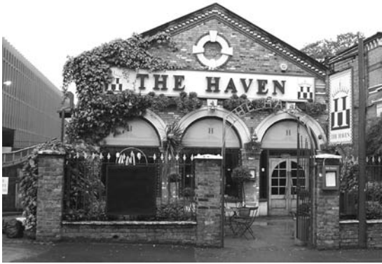
FIGURE 1. This simple building is flexible enough to have served several different functions over the last 30 years, including a bar, workshop, shop, restaurant, and storage.
