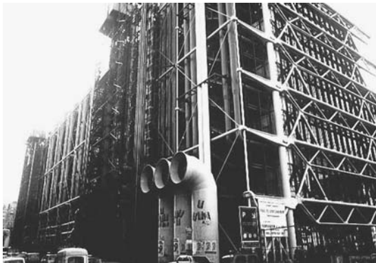
FIGURE 1. Pompidou Centre, Paris.
