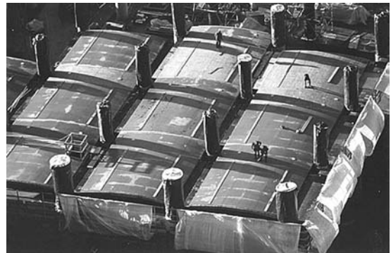
FIGURE 4. Library Square, Vancouver. Concrete Formwork for Exposed Barrel Vault Ceiling.
