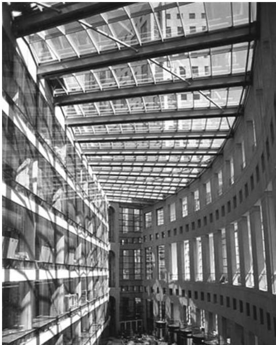
FIGURE 3. Library Square, Vancouver. Skylight and Atrium.
