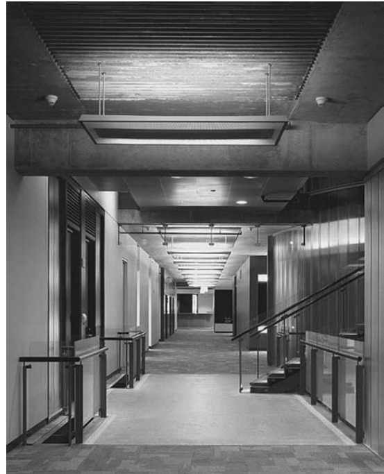
FIGURE 6. Bahen Centre, University of Toronto. Exposed Slab Soffits with Cast-in-place Corrugations.
