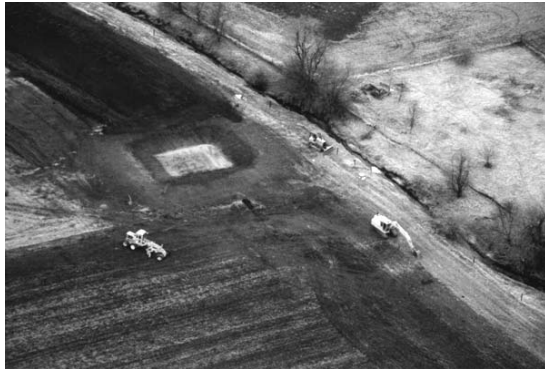
FIGURE 2. Construction of Wetlands.
