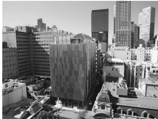
FIGURE 4. Council House 2 (CH2), Melbourne Victoria, the new council building for the City of Melbourne is a 6 Star Green Star rated building with the Australian Green Building Council, the highest rating available in Australia (Designers DesignInc).
