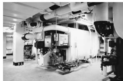
An additional advantage captured by using a gas-fired chiller-heater involved the ability to use waste heat from the absorption process to preheat domestic hot water year-round before the waste heat was sent up to the cooling tower for rejection. In the winter, the waste heat is diverted to the snow melting system at the entrance and exit ramps of the statehouse underground parking garage.
