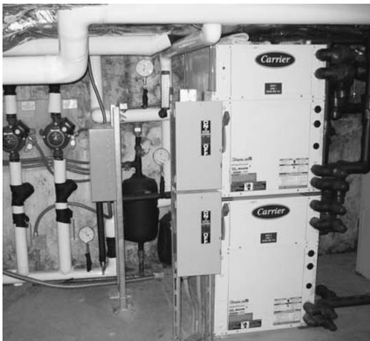
after several years of operation. An environmentally friendly 20% methanol brine solution (with a freeze point of 15°F) is added to the water flowing through the well field to prevent freezing.
