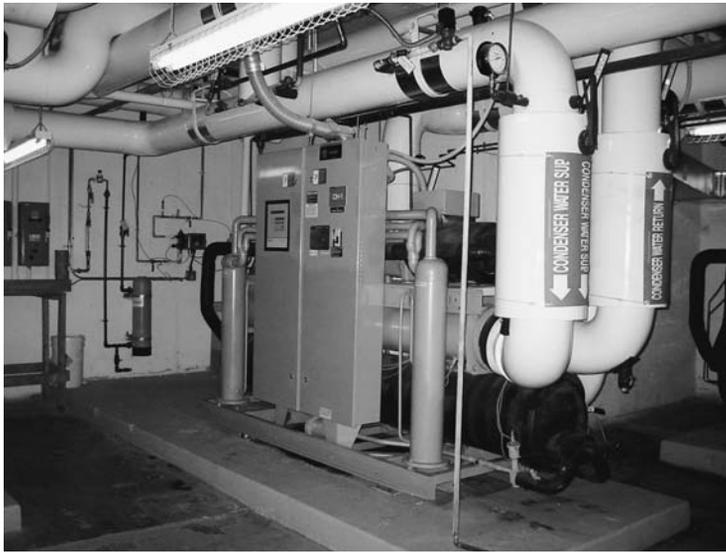
**FIGURE 6.** One of the two 125-ton chillers at the Columbus Museum of Art. Each has the capacity of a 200-ton chiller when used in tandem with the stored ice. (Photo courtesy of Schooley Caldwell Associates.)
