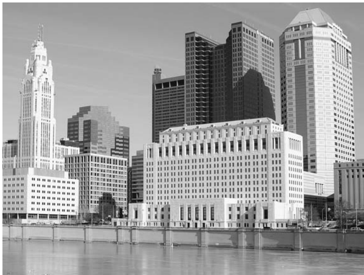
FIGURE 2. The Ohio Judicial Center is home to the Supreme Court of Ohio as well as the state's law library. Limited floor-to-floor heights proved challenging when updating systems. (Photo by Feinknopf Photography.)
