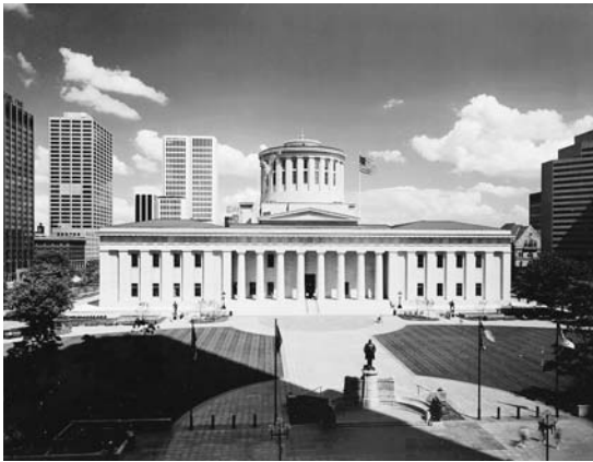
FIGURE 1. The Ohio Statehouse required a complete overhaul of the entire HVAC system, yet had limited space, and as the building is a National Historic Landmark, the new systems and associated equipment had to be incorporated invisibly. (Photo courtesy of Schooley Caldwell Associates.)
