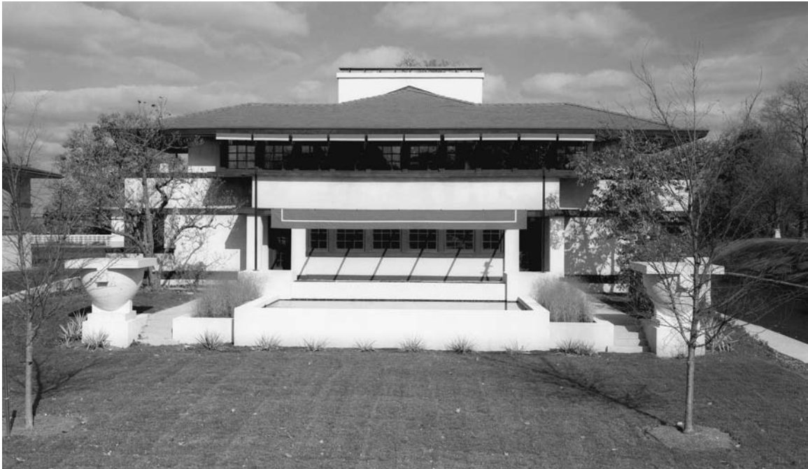
FIGURE 8. Adapting Frank Lloyd Wright's Westcott House into a museum required an HVAC system that would provide a 22-ton cooling load while remaining invisible to visitors. (Photo by Feinknopf Photography.)
