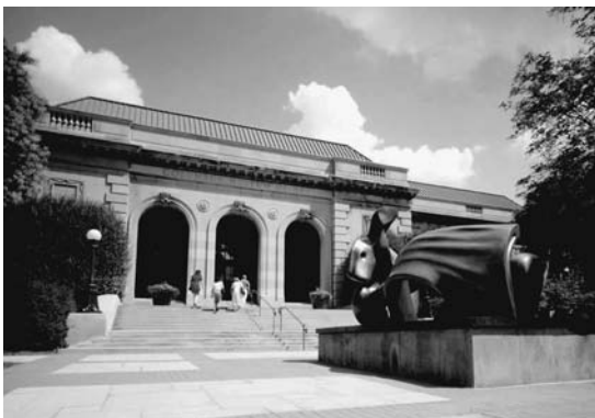
FIGURE 5. The ice storage A/C system at the Columbus Museum of Art allowed approximately a 34–40% shift of peak electrical loads. (Photo courtesy of Schooley Caldwell Associates.)
