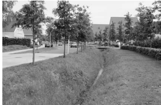
FIGURE 6. Grass swale in Oikos residential development, Enschede, Netherlands.
