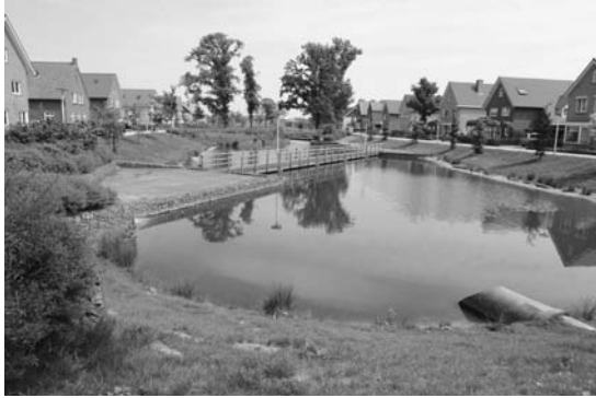
FIGURE 13. Constructed wetland as a central feature in Oikos residential development in Enschede, Netherlands.
