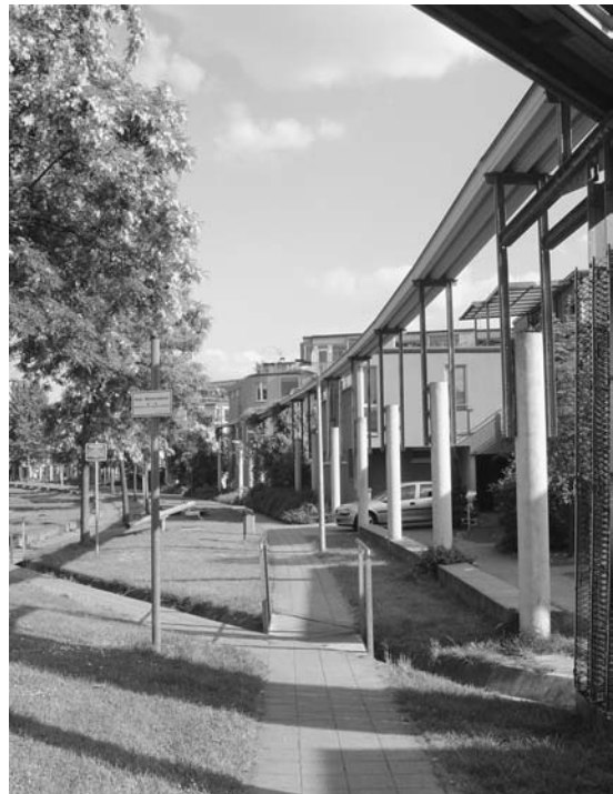
FIGURE 3. High level aqueducts used to collect and transport excess runoff from green roof system, Kuppertsbusch, Gelsenkirchen, Germany.
