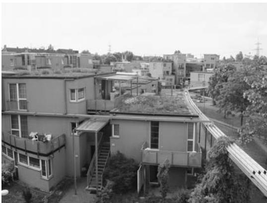
**FIGURE 3.** High level aqueducts used to collect and transport excess runoff from green roof system, Kuppertsbusch, Gelsenkirchen, Germany.
