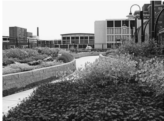
FIGURE 4. Intensive green roof on the Schwab Rehabilitation Hospital designed for both horticultural therapy and recreational use, all within the safety of the hospital grounds. The 10,000-square-foot green roof occupies 50% of the total roof space and has growing medium depths of 8 to 18 inches. The green roof, supplied by American Hydrotech, was the award winner in the Intensive Institutional category at the 4th Annual Greening Rooftops for Sustainable Cities Conference and Trade Show in Boston, MA. Courtesy of Green Roofs for Healthy Cities, www.greenroofs.org .
