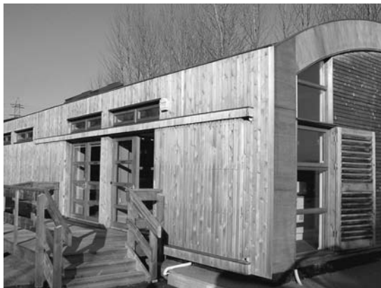
FIGURE 12. The Torfaen Environmental Building.
