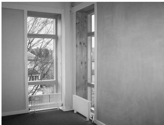
FIGURE 11. ModCell panel finish on interior of Media Center.
