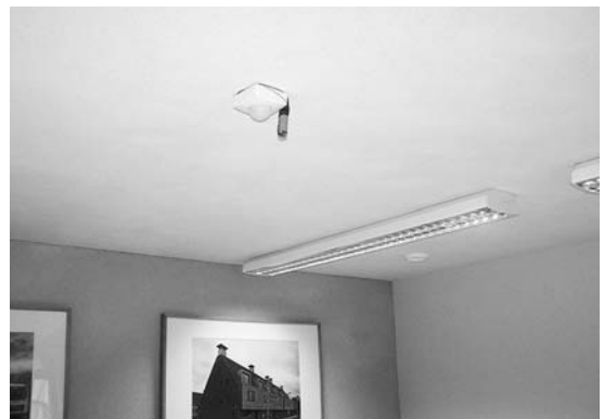
FIGURE 25. Interior of typical office in Lime Technology office.
