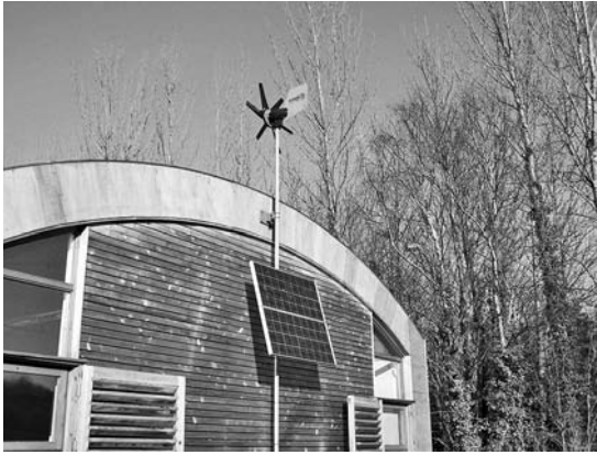
FIGURE 14. Photovoltaic solar panel on Torfaen Environmental Building.
