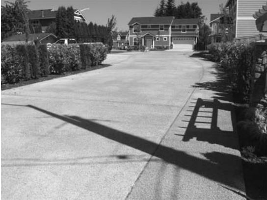
FIGURE 3. Stratford Place in Sultan, WA. All surfaces in the development—streets, sidewalks, and driveways—are constructed with pervious concrete. Colored pervious concrete delineates walkways. Use of pervious surfaces replaced stormwater retention pond, and saved the owner over $250,000.
