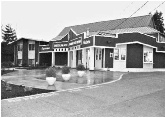
FIGURE 5. Snoqualmie Gourmet Ice Cream, pervious concrete parking area. (AM Photo)
