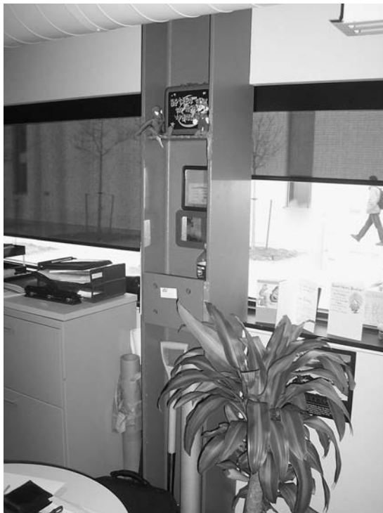
FIGURE 6. The history of the steel was purposefully left visible by not removing the plates and holes from the original use.
