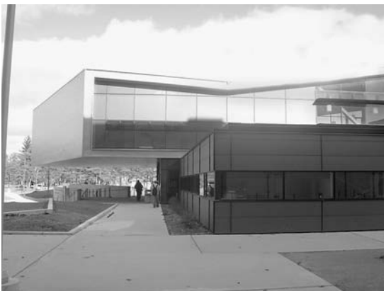
FIGURE 4. UTSC Student centre with reused steel in the lower wing.
