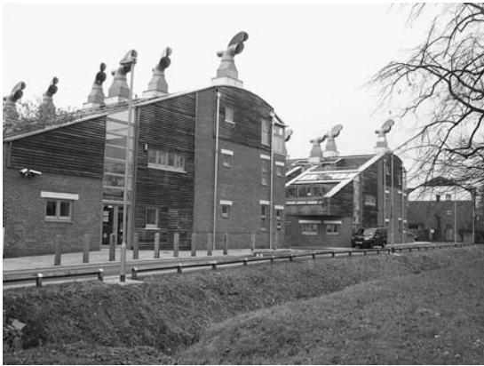
FIGURE 1. The Bedzed development.
