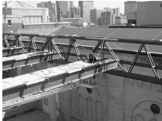
FIGURE 5. Dismantling of steel at the ROM.
