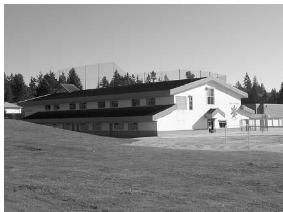
FIGURE 7. The new Roy Stibbs school building featuring reused steel.
