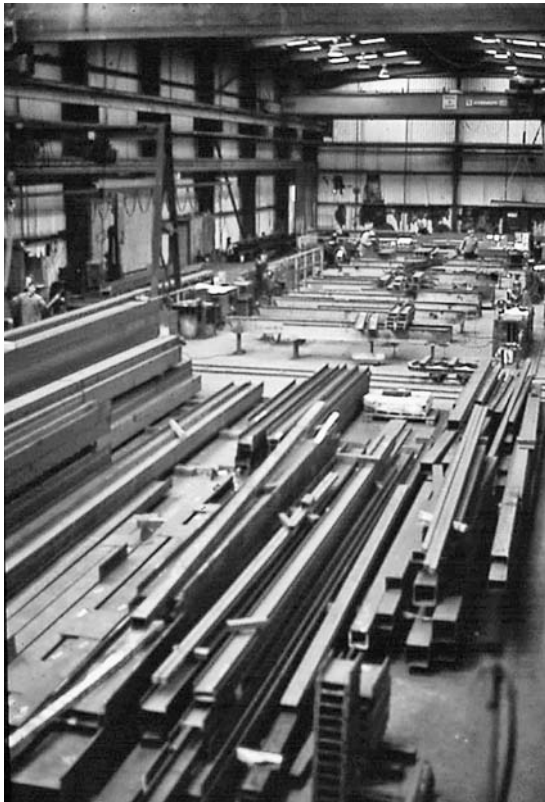
FIGURE 2. Reclaimed steel stored ready for refabrication.
