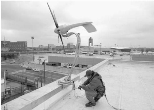
larger turbine. The site at Logan Airport in Boston, MA takes 20 turbines of the type shown above to make the estimated 100,000 kilowatt-hours of energy for the facility to use on-site. A single turbine of 60 kilowatt rated power would be able to do this amount too but would need a 100 foot tower and would have a wingspan of 15 meters (49 feet).
