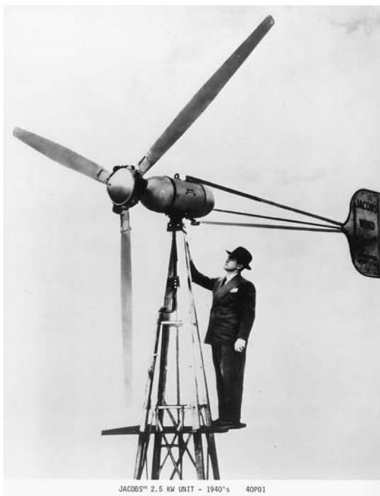
turbines rated voltage, commonly 32 vdc, to work together with the turbines. Also notable in this period was the Jacobs wind turbine, which is still in production today with units to 20 kW.
