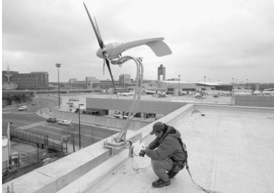
FIGURE 17. AeroVironment installation on building at Logan Airport, this style is called Architectural Wind™ by the company.
