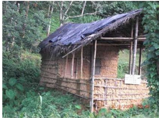
FIGURE 5. Earth walled unplastered peasant house.
