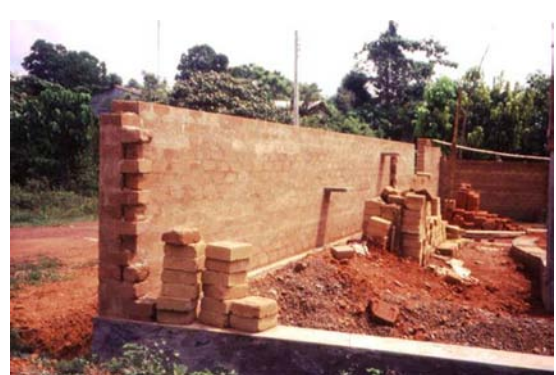
FIGURE 9. Earth walls and bricks at a site.
