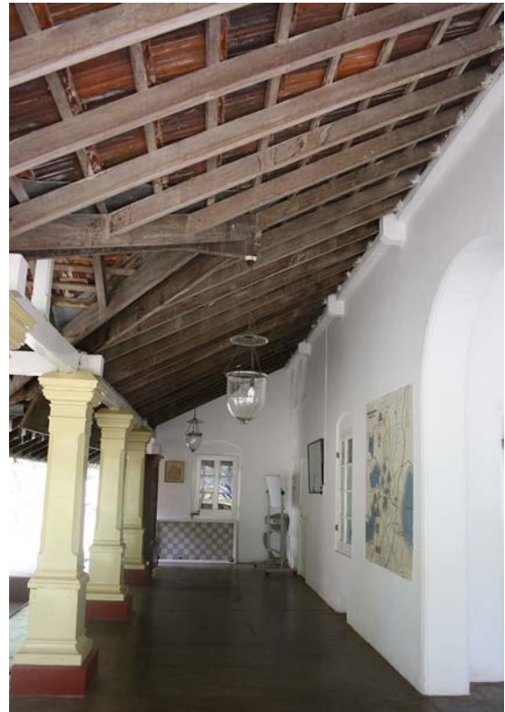
FIGURE 3. Exposed timber ceilings.
