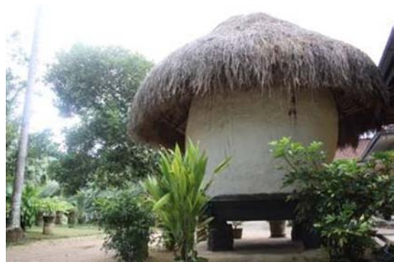
FIGURE 6. Granary Storage houses.
