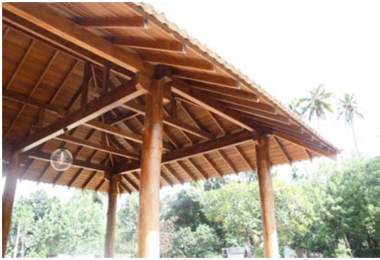
FIGURE 4. Celebrating the exposed timber ceilings.
