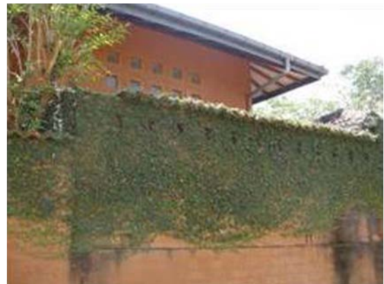
FIGURE 12. Exterior views of the walls: ivy grown over earth walls.
