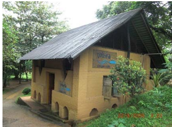
FIGURE 13. Earth cottages in a way-side resort: Ambalama.
