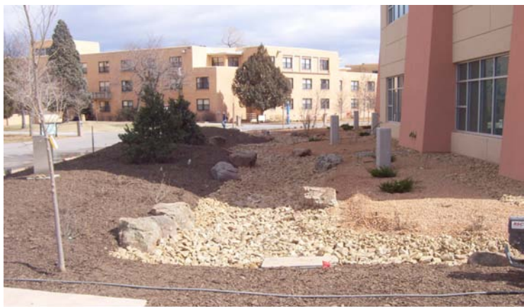
Riverbed landscaping directs and retains water flow.
