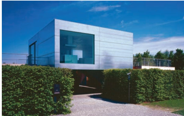
FIGURE 5. Case study 3—“Haus der Gegenwart” in Munich (Germany), using PCM. Image by: F. Holzherr.
