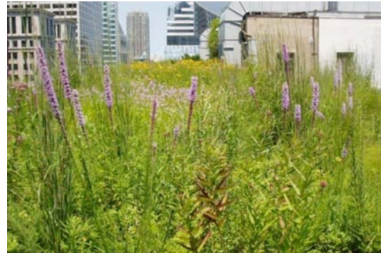
FIGURE 2. Simple intensive green roof system with prairie vegetation on Chicago City Hall Green Roof (photograph B. Dvorak, July 2004).
