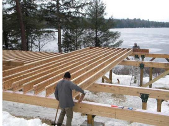
from squaring up our columns and beams; concrete was pumped from the road above; and the crane made its first visit to drop the nearly forty foot long carriers. There was literally no further impact to the site from machinery after this point. Overall, this greatly affected recovery of plantings and access pathways.
