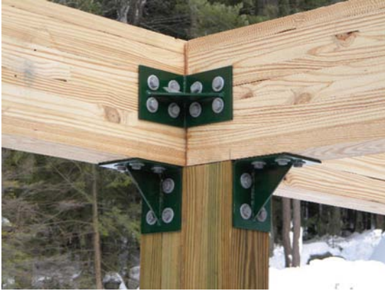
Steel gussets bolted at frame intersections, creating our base frame.
