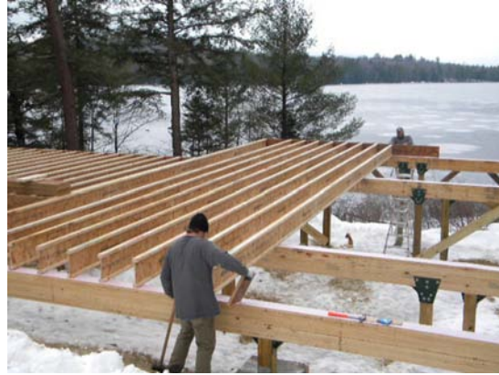
Base frame with continuous joists being placed.
