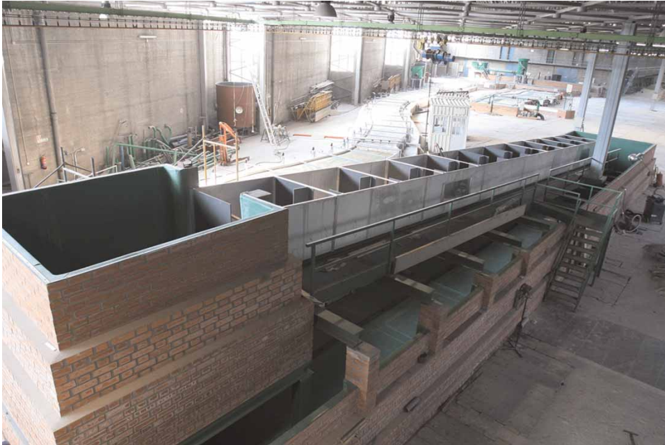
Figure 1 | Full-scale vertical slot fishway model used in this study. Photo taken at CEDEX (Center for Studies and Experimentation of Public Works, Madrid, Spain).
