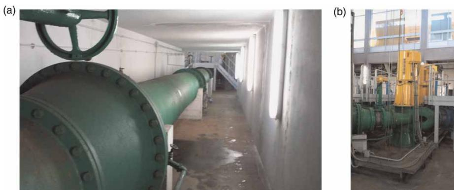
**Figure 2** | Novara pumping station: (a) the pipe inside the station; (b) the pumps.
