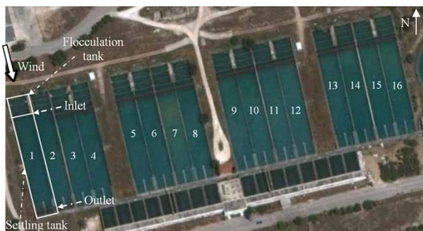
Figure 1 | The settling tanks of the WTPA (obtained from http://www.google.de/intl/de/earth/ ).
