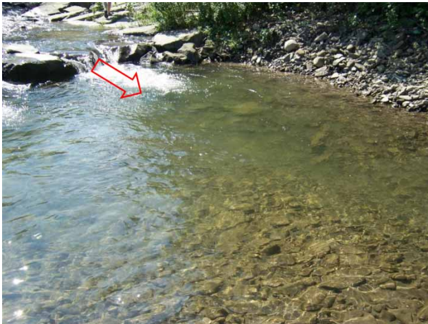
Figure 4 | The scour hole below block ramp on Porebianka stream, Poland.
